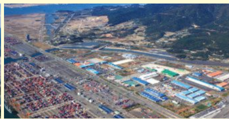
Hinterland of Yeosu-Gwangyang Port
